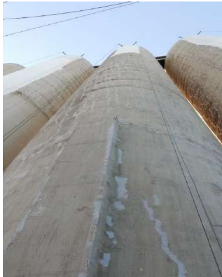
All fissures and cracks filled and area restored
