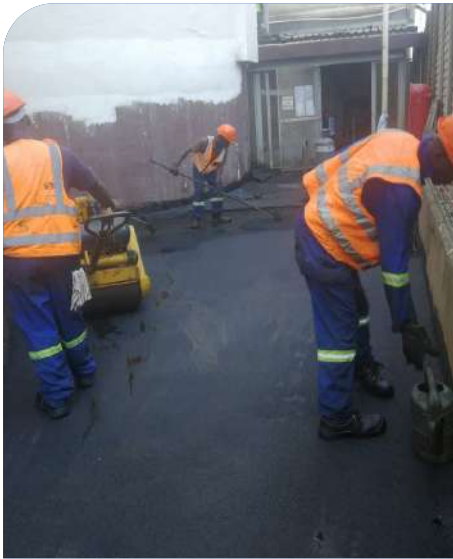
Rescreeded and waterproofed to falls
